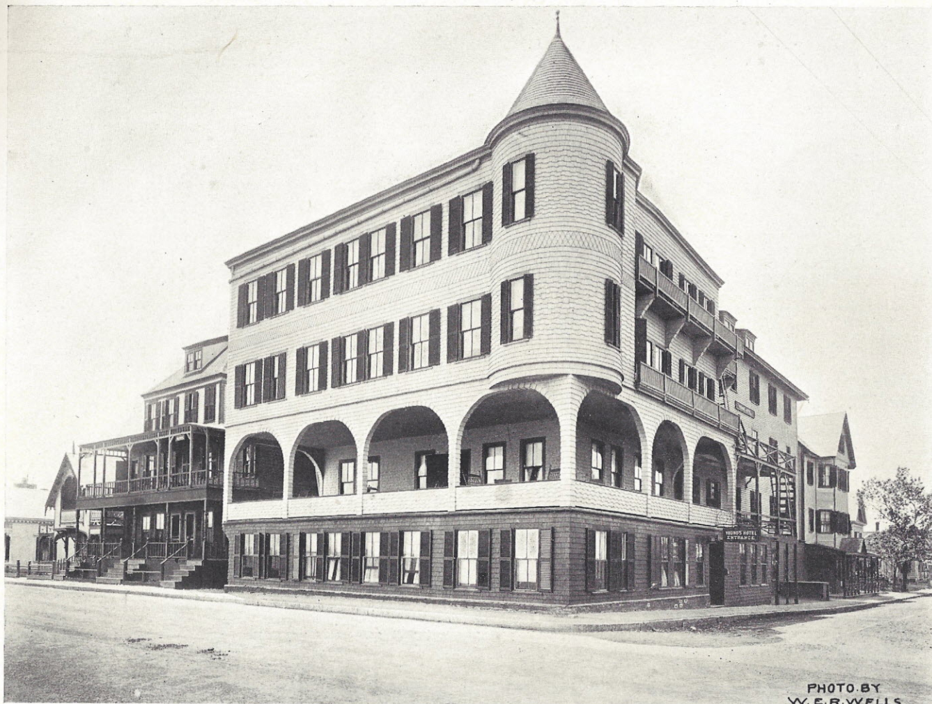
YOUNG'S HOTEL, CREST AVE. AND TEWKSBURY ST.
