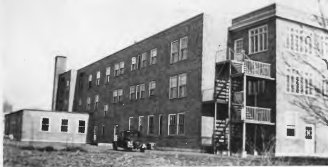
VIEW LOOKING SOUTHEAST TO THE NORTH & REAR OF HOSPITAL.
