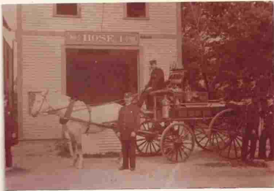
HOSE CO. #1 - FIRST HORSE DRAWN PIECE FOR THIS COMPANY. PLACED IN SERVICE JUNE 1, 1891
