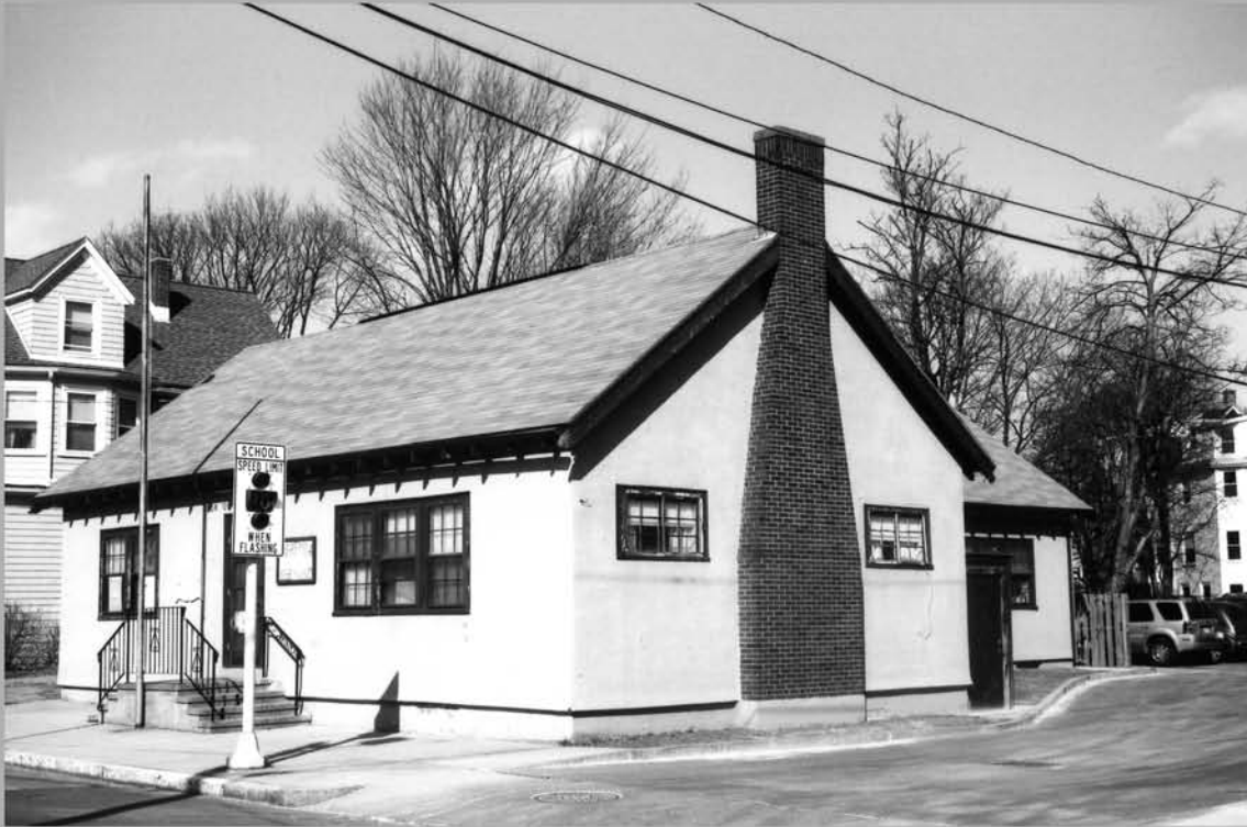
21A. 29 Hermon Street, former American Legion Hall
