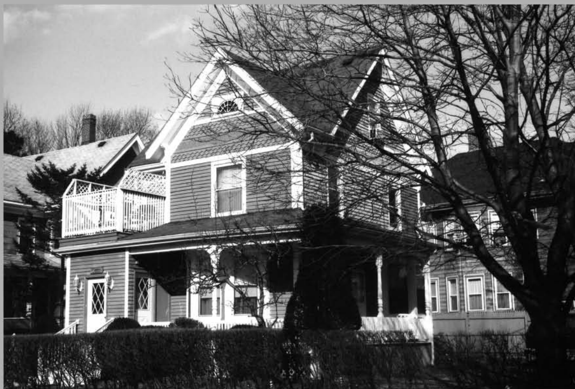
16A. 100 Fremont Street, Belcher-Nickerson House
