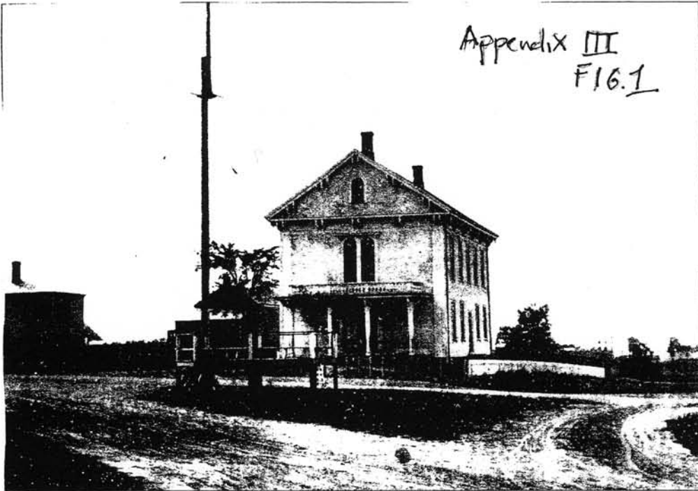
Winthrop's original town hall, built in 1856, occupied the corner of Metcalf Square where the old post office was and where the new police station now stands. The first floor was devoted to two schoolrooms and town offices, while town business was conducted on the second floor. The total cost of this building was $4,990 and served the town well until the present town hall was erected in 1929. Note the bandstand in the center of what is now the square.
